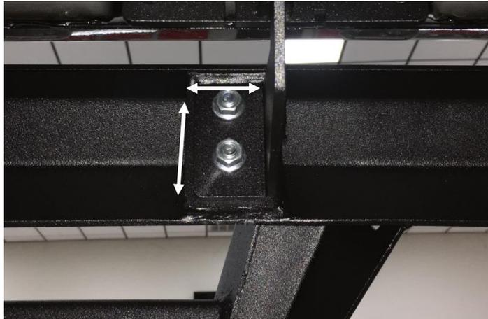
**Step 7:** After final positioning, begin at the rear bracket and tighten the lower bolt to 15-20 ft. /lb. Continue to the front bracket and then to the center bracket. Next, tighten the upper mounts from front to back at 15-20 ft. /lb.
