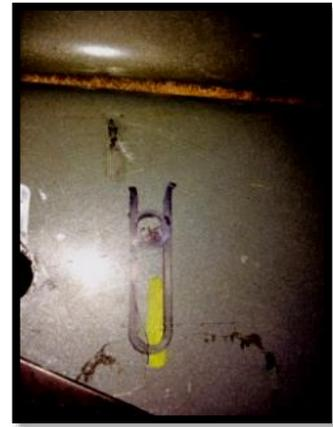
**Step 8:** Remove clip. Use a 1/2” drill bit and drill out the center mark. Slide the 3/8 clip back into position so the threaded part is aligned with the hole.
