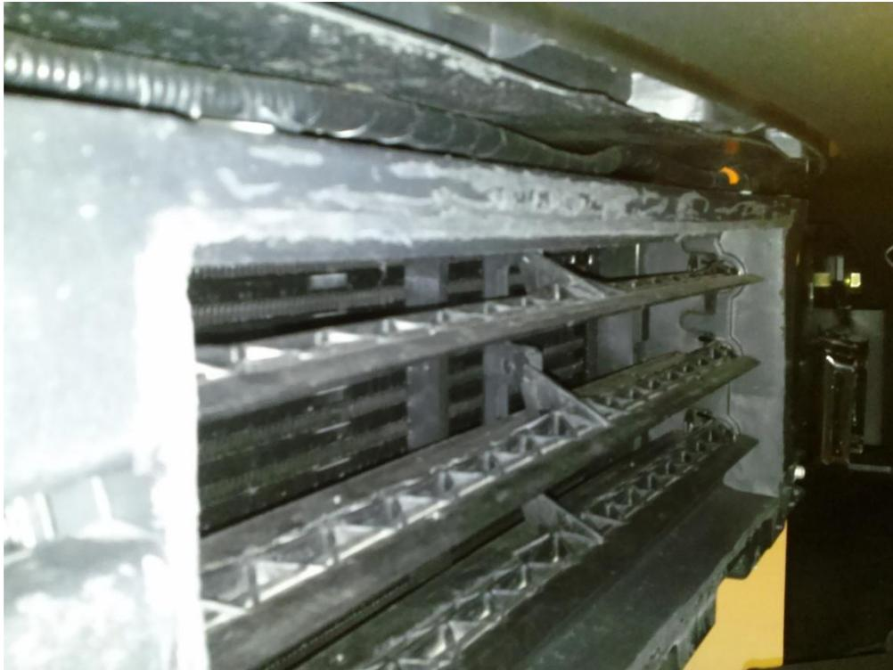
**Figure 4 (Louver w/ shroud cut away at base)**
